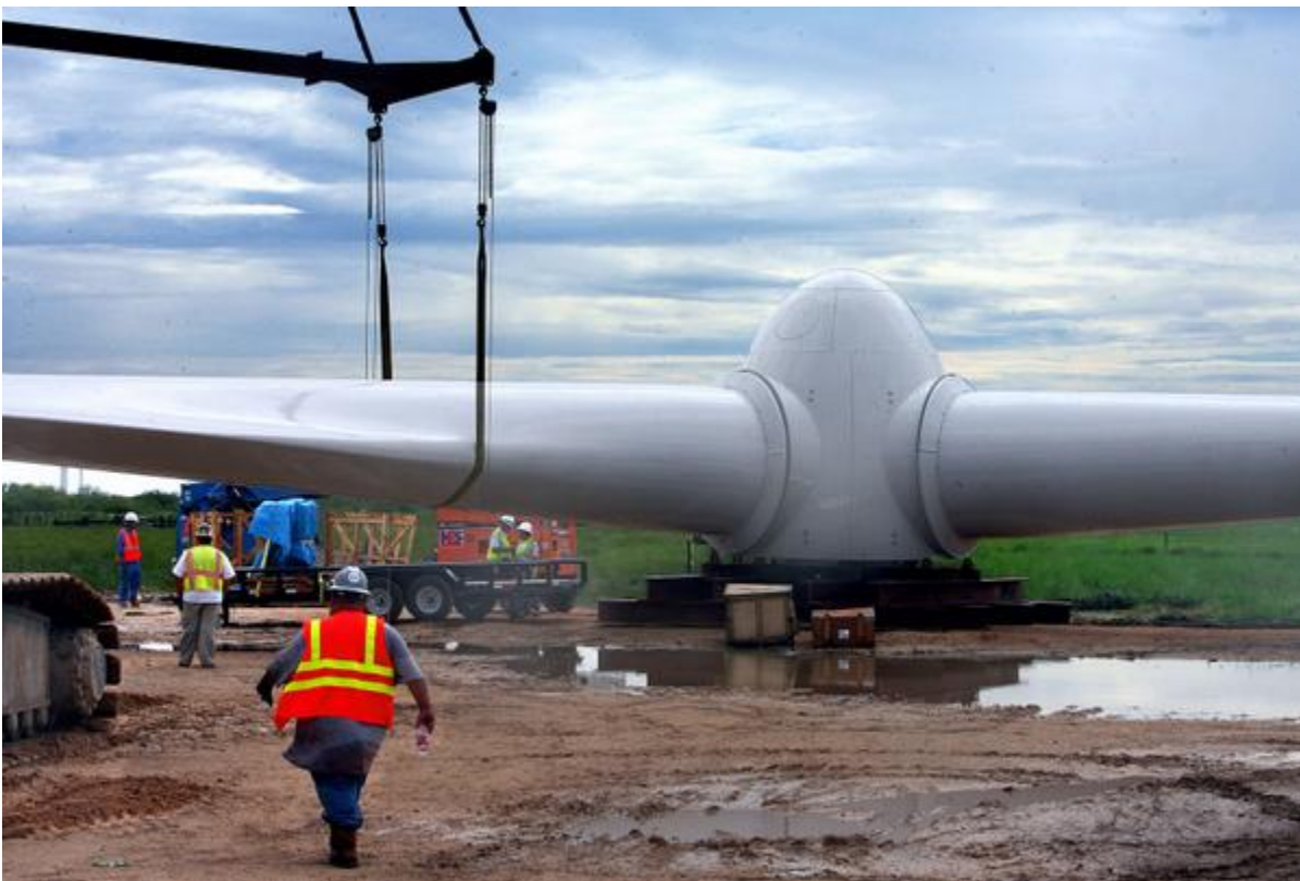
Photos by George Gongora/Caller-Times Workers prepare to hoist part of a giant turbine at the Penascal Wind Farm south of Sarita on U.S. Highway 77. As of Tuesday, four of the farm's 118 turbines had been erected. Each turbine blade weighs more than 12 tons.
